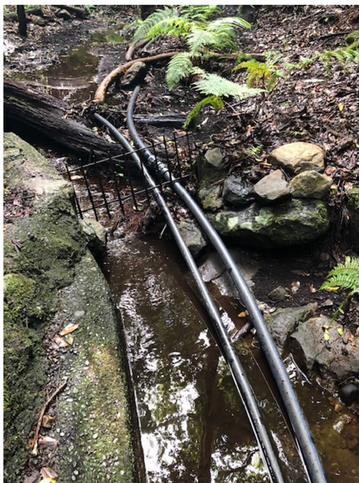
Figure 5. Drainage of Meriga (La Gomera) stream water by means of open canal and pipes (V. Lüderitz).
